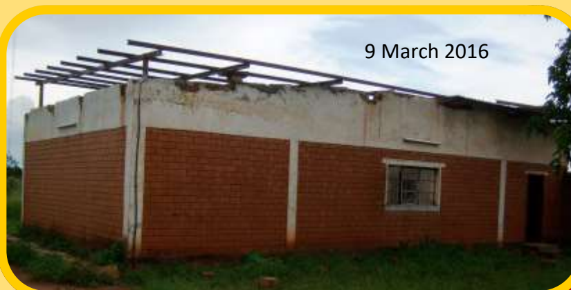
The new iron support poles and iron beams are in place, ready for red oxide then the new roof.
