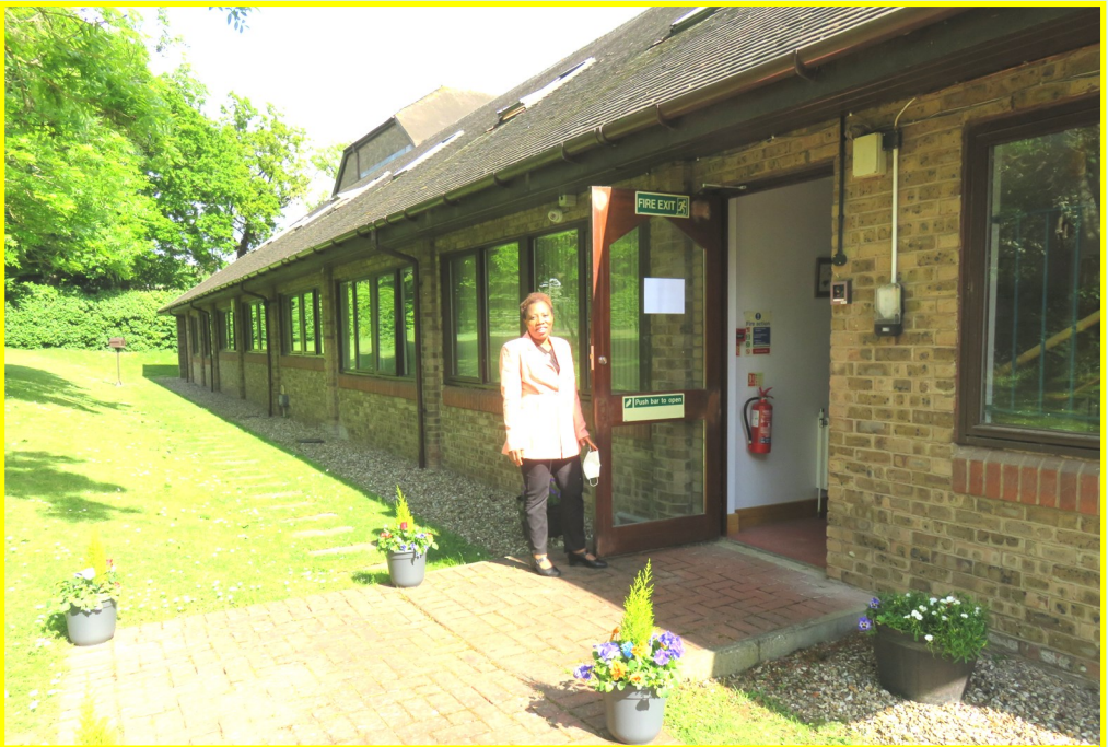
A new entrance has been created for visitors of the lay residents to allow a little more privacy for the Sisters.
